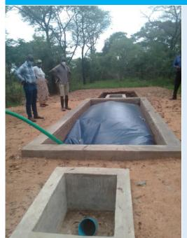
The biogas systems are to be fed with waste daily to avoid any glitches in functionality. Waste fed includes any bio-degradable waste around the household and other livestock waste including chicken waste. The biogas systems have a heating capacity for 5 000 chickens.
