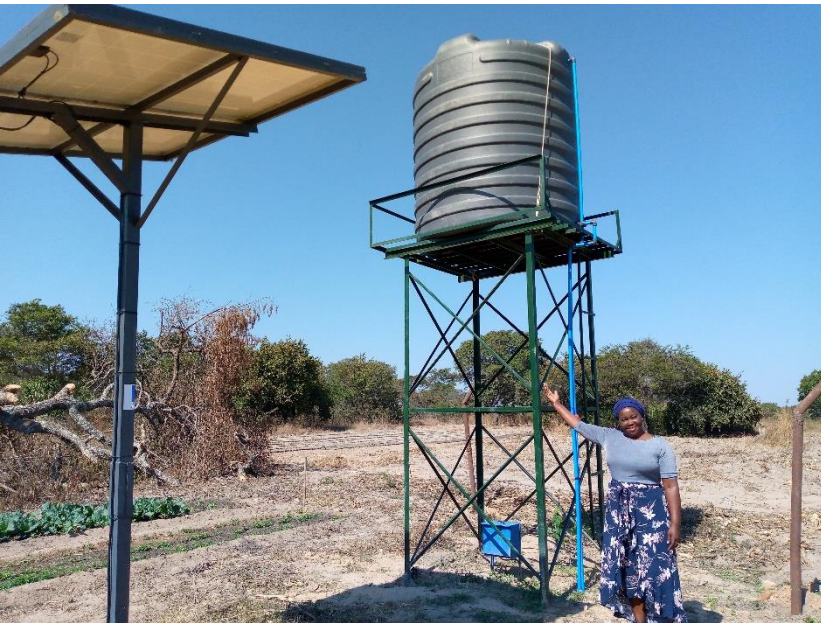
Marwa installed a solar powered water pumping system and a 5,000 litre water tank for watering her dairy herd and irrigating pastures.
