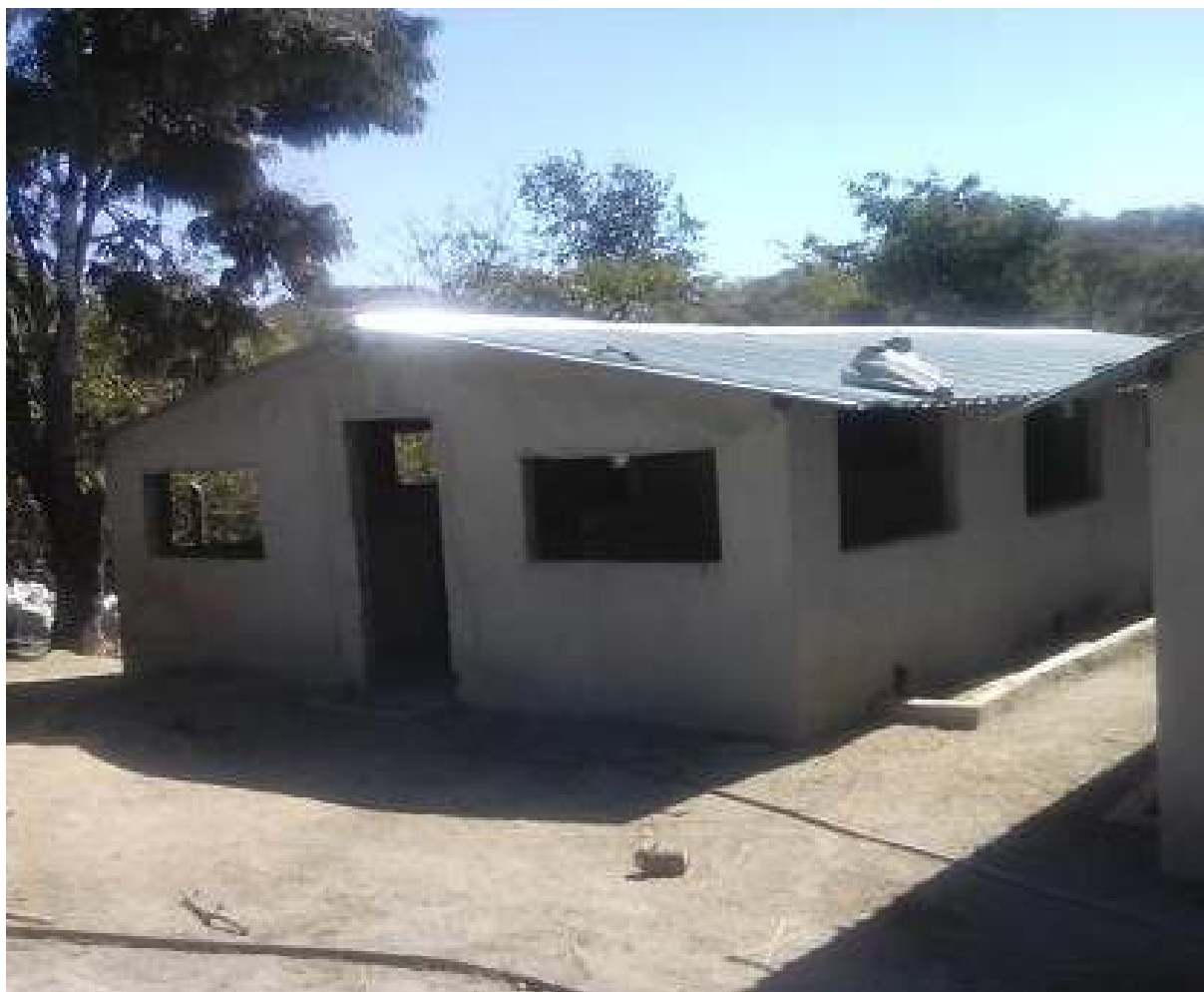
Figure 6-3 Cement plastered brick walls
