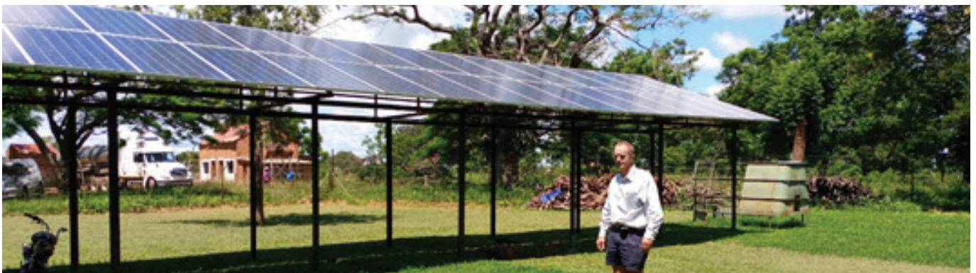
The Matching Grants Facility (MGF) has enabled dairy enterprises to invest in productive assets and infrastructure. John Crawford from Portlet Farm in Makonde district in Mashonaland West Province showing the solar system acquired through MGF and installed at the Farm to power milk cooling tanks.
