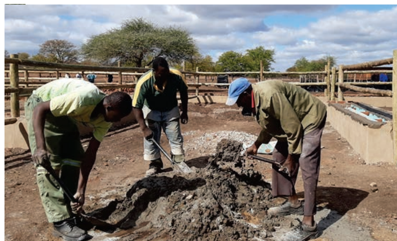
Figure 8: Youths in Chiredzi employed to construct the Cattle Business Centre (CBC)
